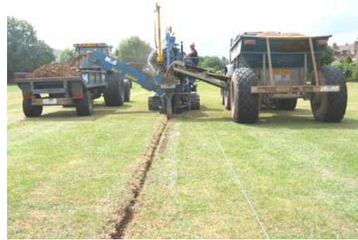
The Drainage Team installing pipe for Haberdashers College, London.
