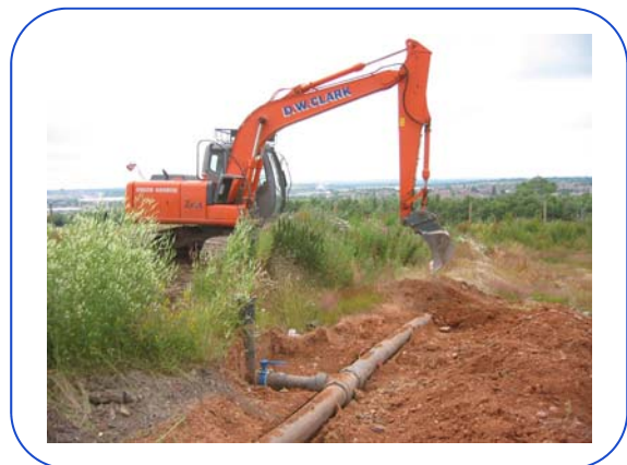
Back filling a newly installed pipe connection at Poplars.
