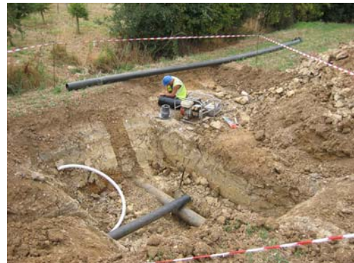
Preparation for main line connection at Roxwell site.
